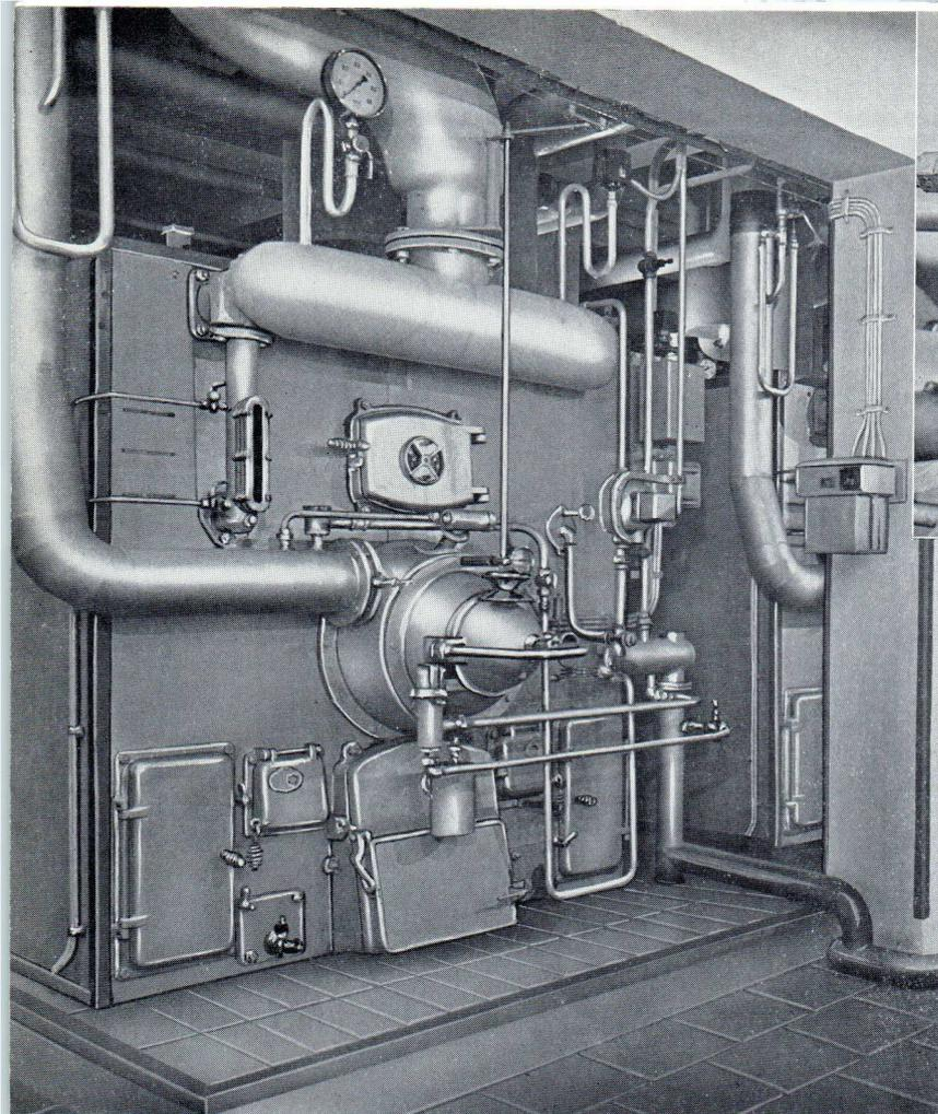
*Flame control with phototube. A phototube „watches” the fire in the boiler. When the fire extinguishes the fuel supply is stopped and an alarm signal is given, so explosion is prevented.*
