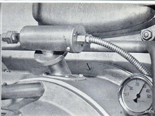
*Mounting of the phototube holder on the boiler. The tube is protected against possible damage by cast iron container.*
