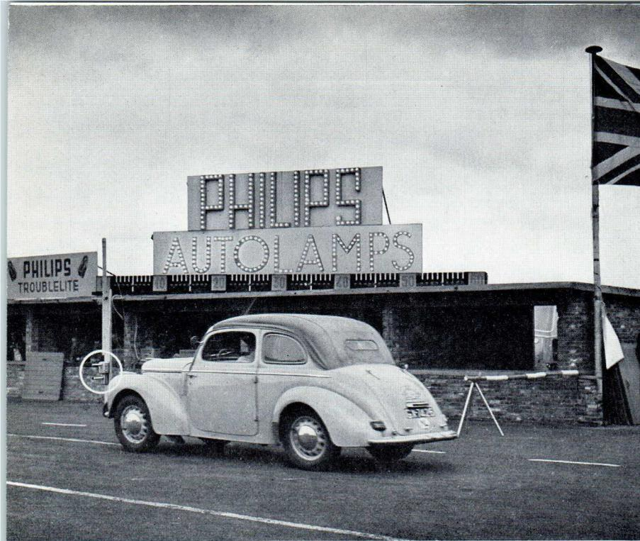
*Accelerating contest for motor cars. The car starts at a given point and at the starting signal lamps are successively automatically lit behind the time scale on the stand. Each second is counted. The counting mechanism stops as soon as the motor car passes the line from the light projector to the phototube and the public can easily read the time made by each car.*
