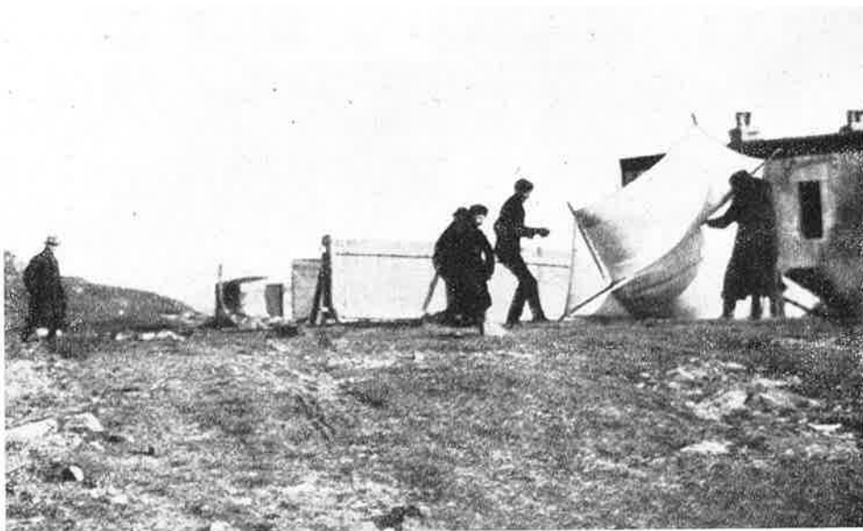
Across the Atlantic, Marconi and associates erecting a kite-supported aerial to receive transmissions from the high-power station in England.
