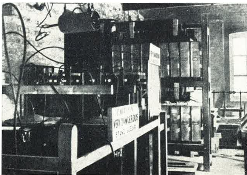
Part of the transmitting apparatus at Poldhu with which the first signals were made across the Atlantic.
